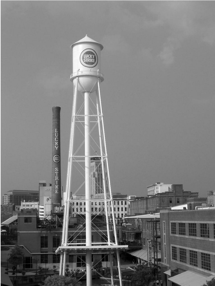
Figure 5: Smokestack and water tower at the American Tobacco Campus. Courtesy of LearnNC.org.
